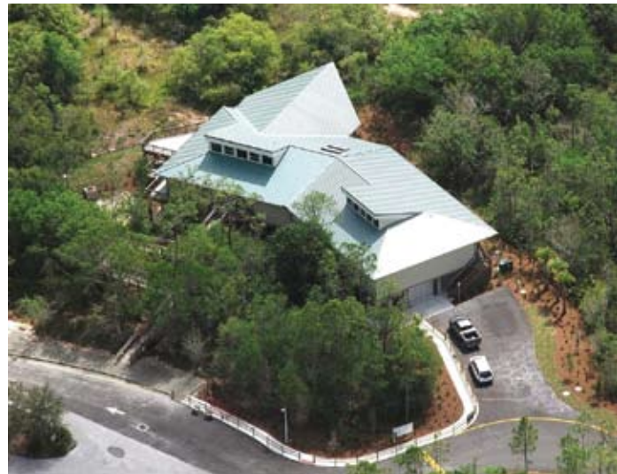
Eagle-eye view: An aerial photograph of the Interpretive Center at Six Mile Cypress Slough Preserve shows how few trees were removed during construction.
